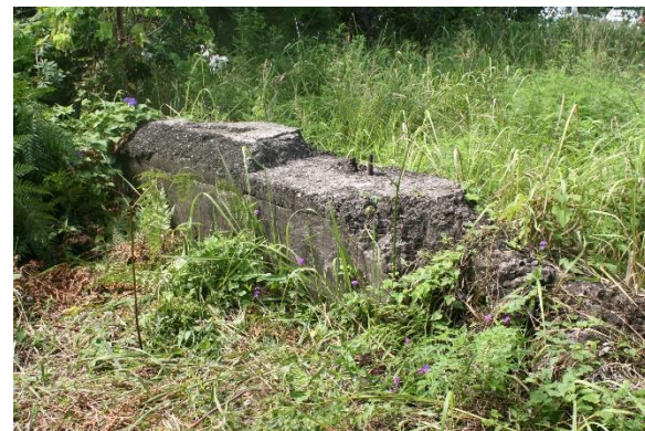
Plate 6. Former concrete structure.
