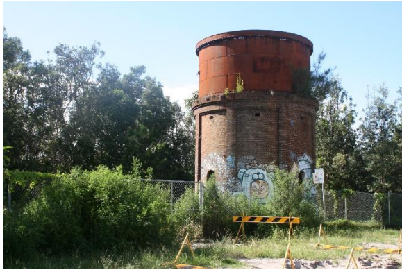
Plate 1. Water tower within the subject area.
