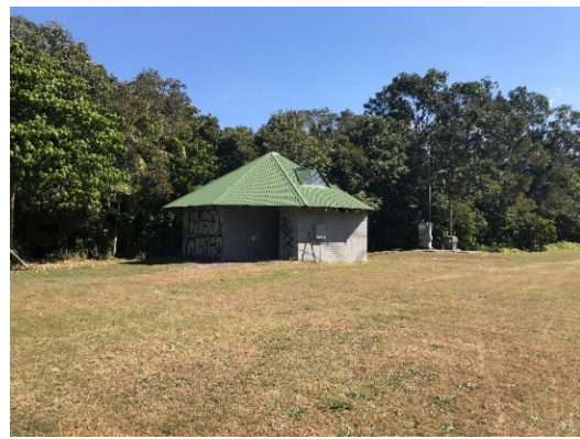
Figure 35: Toilet Block located at the end of Somerset Street
