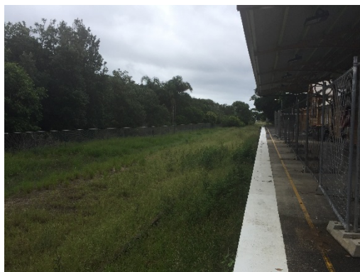
Figure 19: Railway Corridor on existing platform looking north northwest
