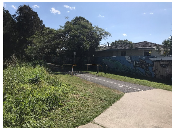
Figure 30: Butler Street bridge over tributary of Belongil Creek looking towards Shared path
