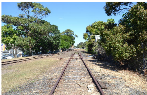
Figure 20: Railway Corridor looking South from near Shirley Street
