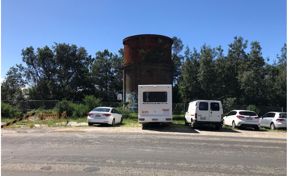
Figure 46: Viewpoint 5 – Existing view from Butler Street looking east
