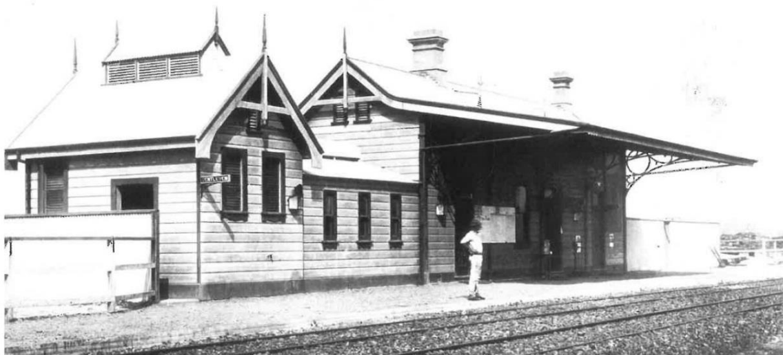
Figure 12. Byron Bay station circa 1896. Note the rail track is at building level and the Refreshment Room has not been added. (Source: NSW Railway Archives; reproduced in Byways of Steam , op cit).
