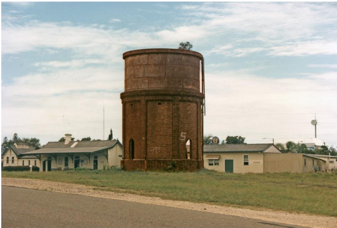
Figure 26. Byron Bay Railway Station in the 1970s, viewed from the south-western (Butler St) with the water tower in the foreground. Note the cleared and level nature of the Loco Siding area. (Source: EJ Wright Collection – Richmond Tweed Regional Library).
