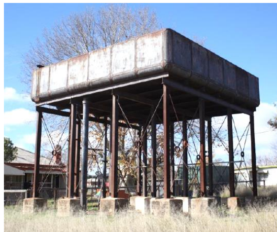
Figure 61. Early type rectangular railway water tank (l) and the later, more common type of railway water tank (r) (Source: Watering Facilities Report op cit)
