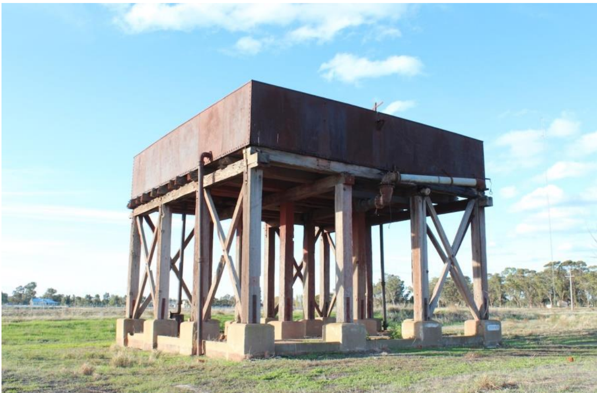
Figure 32. Early style of metal-plate water tank used on the NSW Railways (Source: Extent Heritage).
