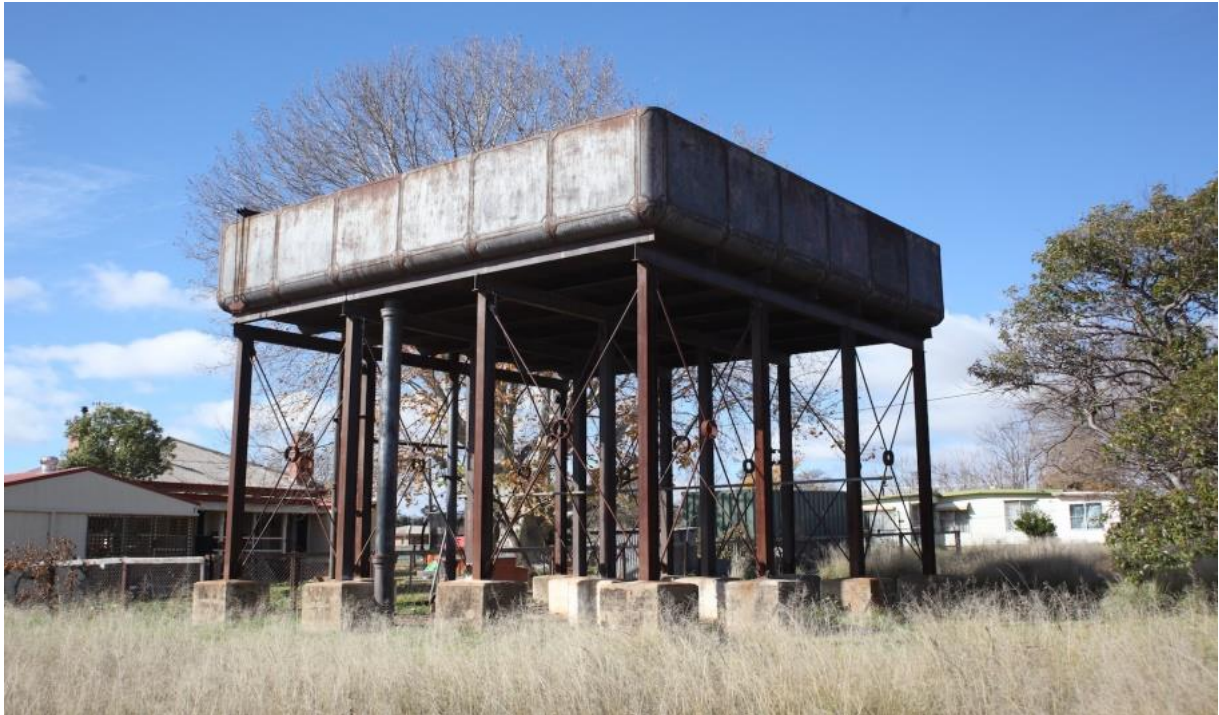
Figure 33. Later style of metal-plate water tank used on the NSW Railways (Source: Extent Heritage).
