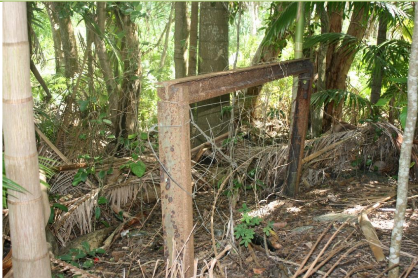
Figure 59. A small section of fencing constructed with pieces of old rail. It is impossible to determine the age and origin of this fence.
