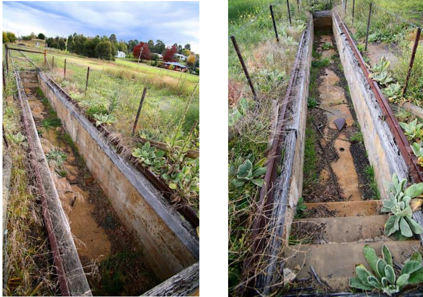
Figure 25. Ash Pit surviving and exposed at Bombala railway station. (Source: P. Buckley; http://sydneyrailwaystations.wordpress.com/ ).
