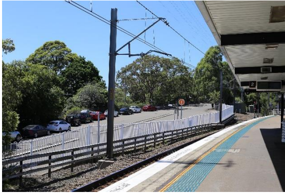
Photograph 11 Rail corridor and Railway Road interface
