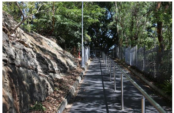
Photograph 14 Rock cutting to pedestrian entry ramp
