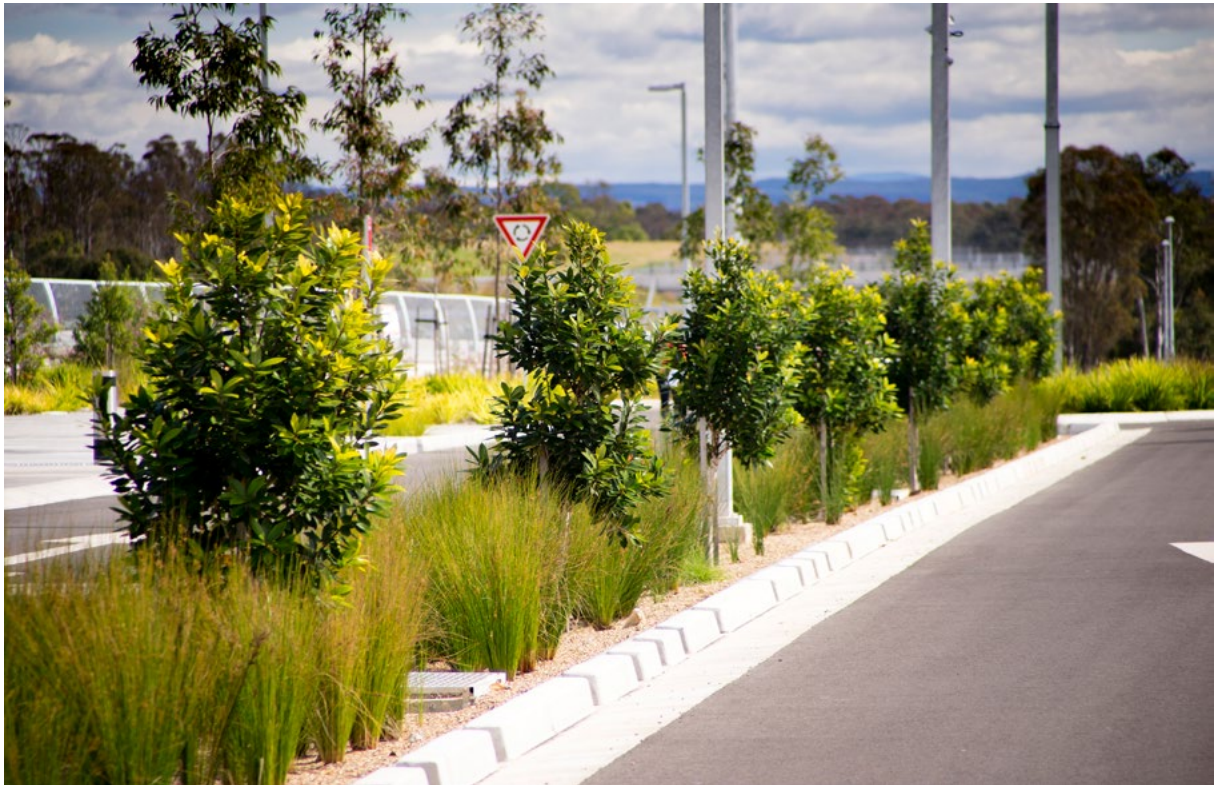
Bio-retention garden beds (raingardens) at Leppington Station car park which remove pollutants from stormwater before it enters local waterways.
