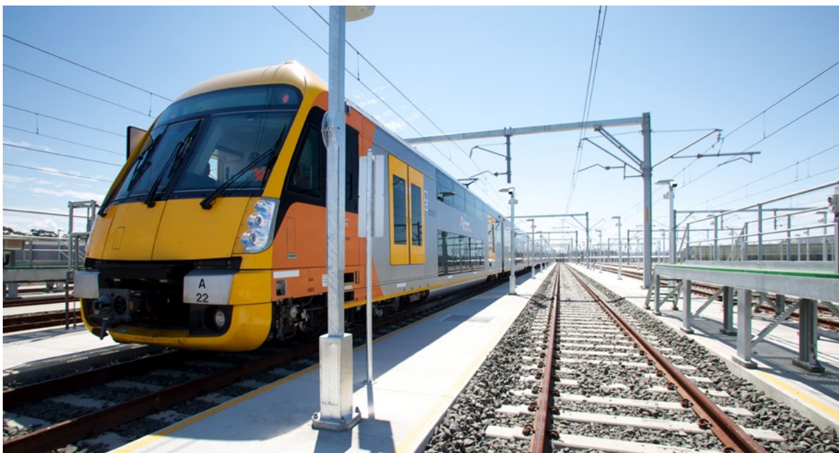
Auburn Stabling Yard – as much of the site was contaminated, spoil was kept on site and capped rather than taken to landfill.
