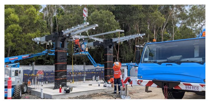
Amenities Block - Structural Steel Erection, October 2020.
