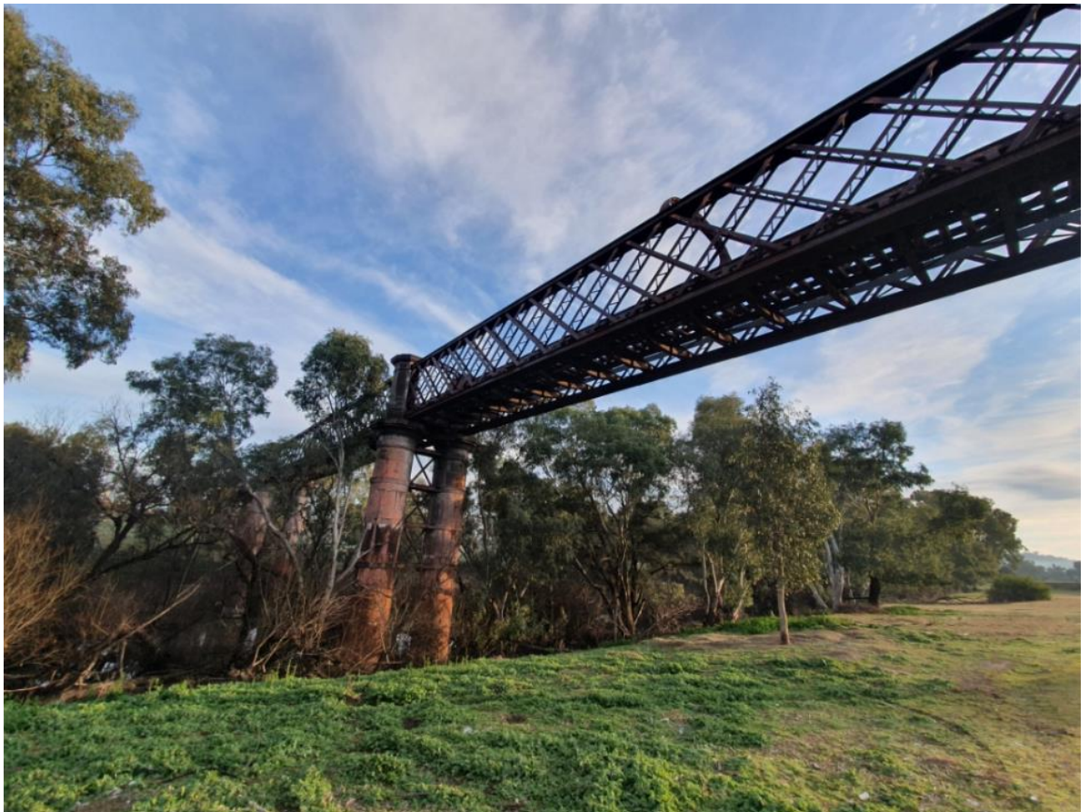
Figure 2 – Cowra viaduct iron lattice spans
