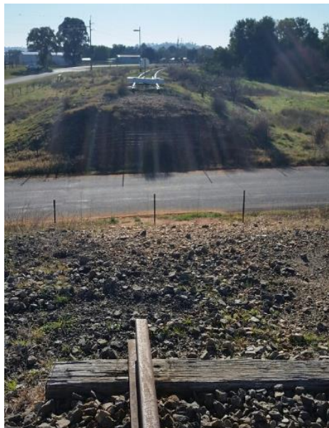
Figure 6 – Underbridge cut at Bulkhead Road Cowra (369.5km)
