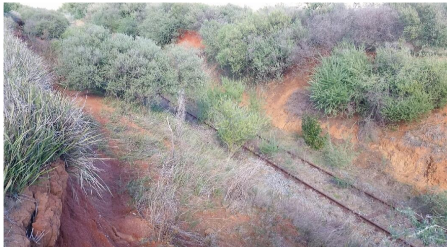
Figure 5 – Cutting with significant vegetation (approximately 447km)
