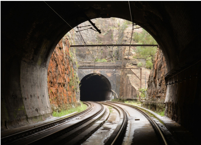
Ten Tunnels Deviation, February 2019
