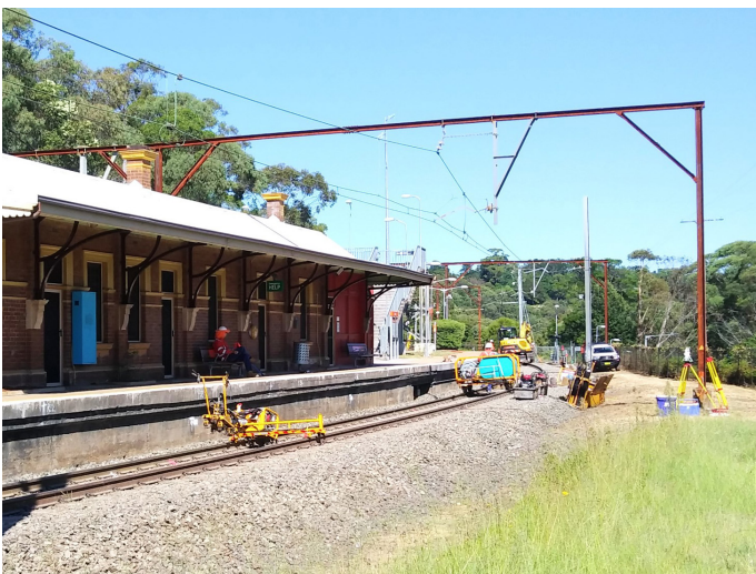
Work at Linden Station, February 2019
