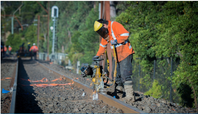
Trackwork on Blue Mountains Line, May 2019
