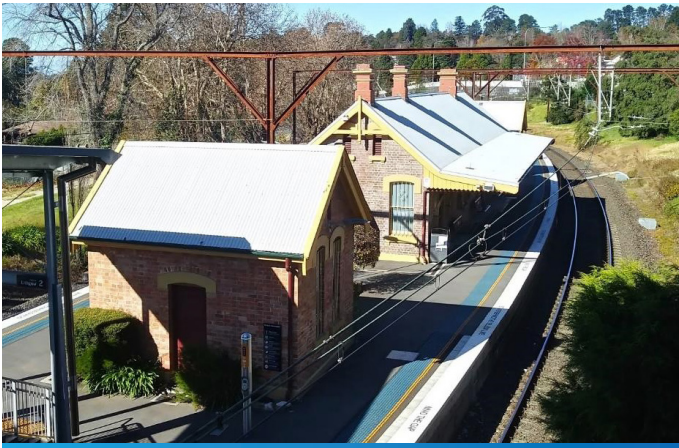
Wentworth Falls Station, May 2020
