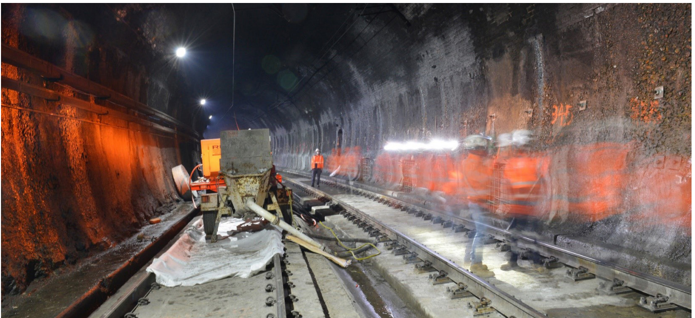
Work in the Ten Tunnels Deviation, September 2019
