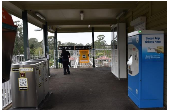
Figure 56: The entrance to the station along the footbridge, view south-east (Source: Artefact 2021)
