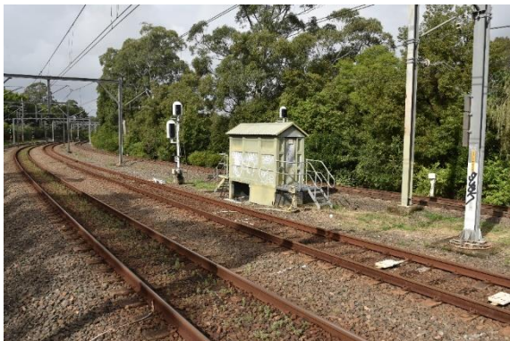
Figure 95: The signal box as viewed from Platform 1/2, view south (Source: Artefact 2021)
