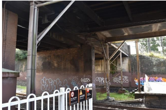
Figure 42: View of the south-western sides of the brick piers and additional steel supports (Source: Artefact 2021)
