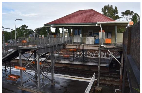
Figure 58: The steel support structure of the footbridge and staircase (Source: Artefact 2021)
