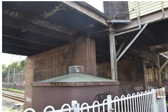
Figure 42: View of the south-western sides of the brick piers and additional steel supports (Source: Artefact 2021)
