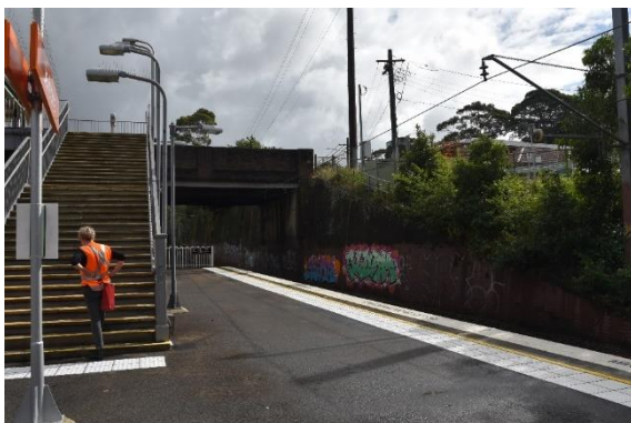
Figure 91: The north-eastern retaining wall from Platform 1/2, view north (Source: Artefact 2021)
