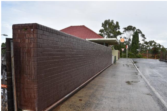
Figure 37: View north-east along the overbridge (Source: Artefact 2021)
