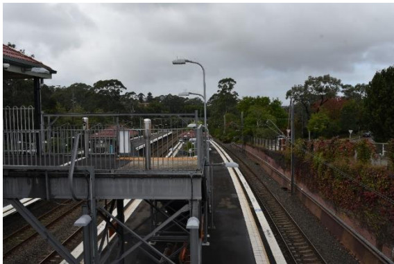
Figure 55: The south-western end of the footbridge, view south-east (Source: Artefact 2021)
