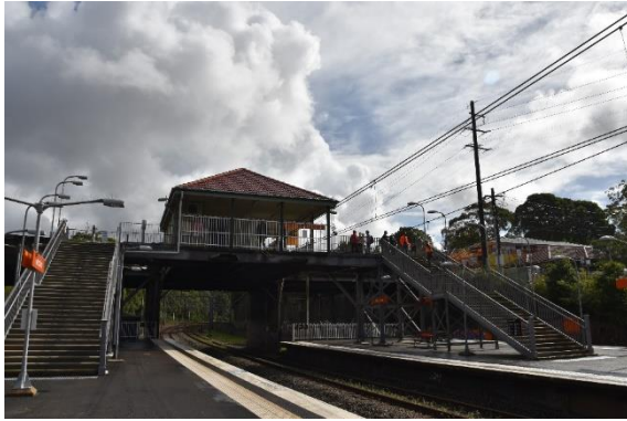
Figure 53: View of the footbridge from Platform 3/4, view north (Source: Artefact 2021)
