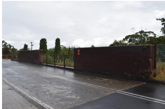
Figure 38: View west to the north-western side of the overbridge (Source: Artefact 2021)
