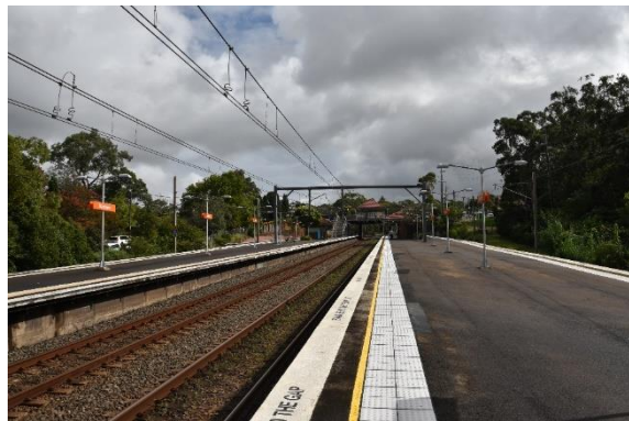
Figure 82: The platforms from the staircase on Platform 3/4, view south-east (Source: Artefact 2021)
