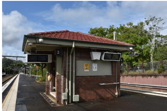
Figure 78: The north-western elevation of the Shelter Shed on Platform 3/4, view south-east (Source: Artefact 2021)
