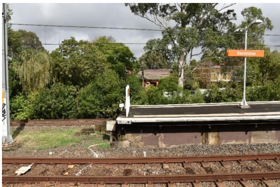
Figure 87: The south-western end of Platform 3/4, view south-west, showing the concrete staircase (Source: Artefact 2021)
