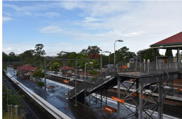
Figure 54: View of the footbridge and staircase to Platform 1/2 from the overbridge, view south-east (Source: Artefact 2021)
