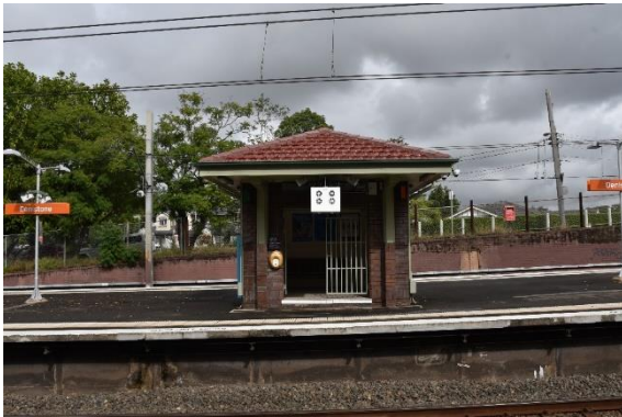
Figure 77: The front (north-eastern) elevation of the Shelter Shed on Platform 3/4, view south-west (Source: Artefact 2021)
