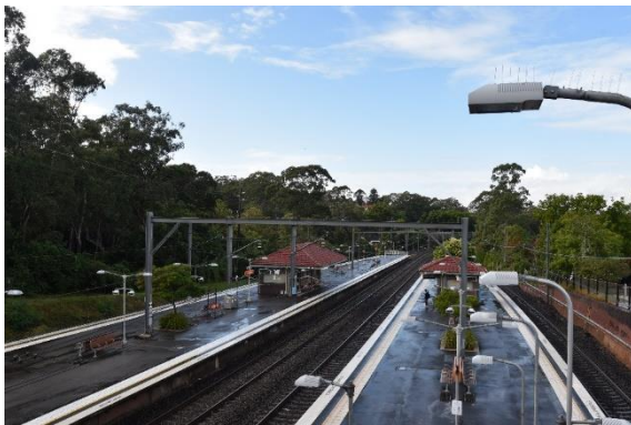
Figure 81: The platforms from the staircase on Platform 3/4, view south-east (Source: Artefact 2021)
