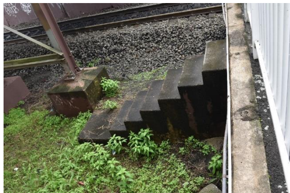
Figure 88: The north-eastern side of Platform 1/2 from East Parade, view north-east (Source: Artefact 2021)
