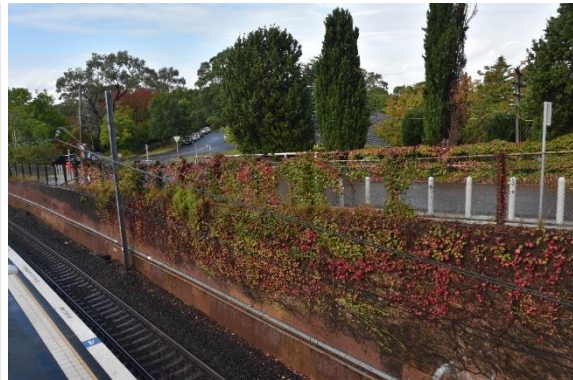
Figure 94: The south-western retaining wall from the footbridge, view south (Source: Artefact 2021)
