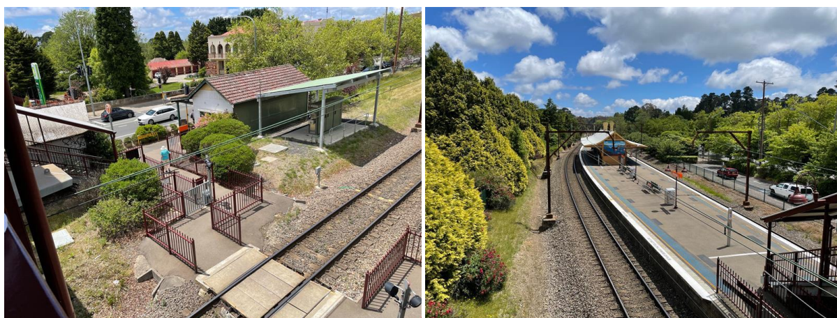
Photo 4.1 Blackheath Station and railway line
