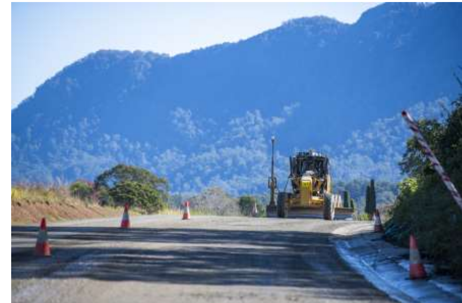
Work between Pumpstation to Fernridge, east of Bellingen
