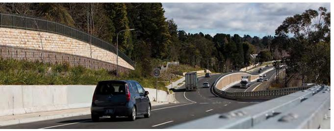
Figure 3.15 Smooth top edges of retaining walls provide a flowing character as seen near Wentworth Falls. Source: RMS.
