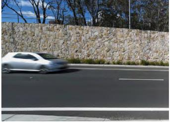
Figure 3.20 Informal pattern of a sandstone clad retaining wall along the Great Western Highway.
