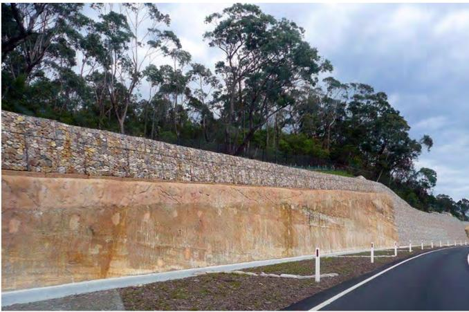
Figure 3.14 Sandstone gabion baskets complement the geology of the area in situations of cuttings as seen in Boddington Hill, Great Western Highway.
