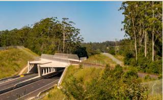
Figure 4.25 Example of a railway and highway bridge interface with a strong skew. Pacific Highway at Warrell Creek
