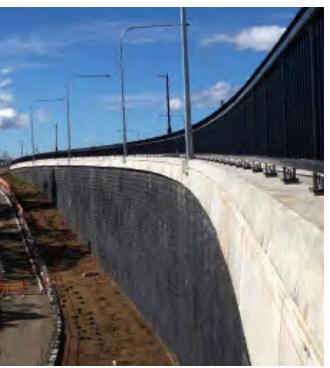
Figure 3.23 This section of the Great Western Highway at Woodford to Hazelbrook illustrates the typical treatment for retaining walls facing away from the highway.
