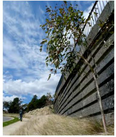
Figure 3.13 Dark receding colours are recommended for walls facing the bush as seen in Den Hogan Drive, Leura. Photo credit: Catherine Dung.
