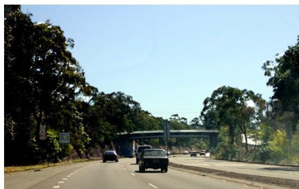
The vehicle overbridge at Fletcher St (western Glenbrook) marks the boundary between Glenbrook and Blaxland. Few other distinctive built features occur along this length, however the scale and density of trees is impressive.
