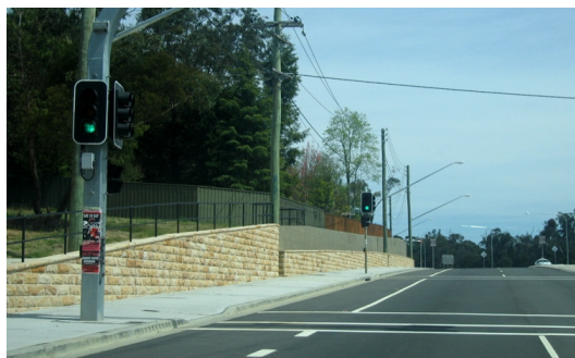
New split level sandstone retaining walls at Mitchell St.
