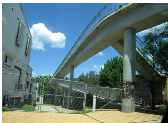
The ramps and associated landing areas however, present an awkward resolution, due to less than adequate space made available for the ramp and partly due to a clutter of other street side elements in their immediate vicinity.
