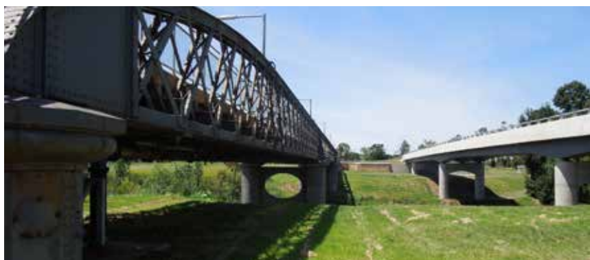
^ THE NEW ROAD BRIDGE AT ABERDEEN PROVIDES A STREAMLINED ELEGANT STRUCTURE THAT VISUALLY COMPLEMENTS AND IS SYMPATHETIC TO THE HERITAGE BRIDGE, WITH PIERS THAT ALIGN IN PLAN, A ROUNDED PIER SHAPE THAT IS SIMILAR TO THE HERITAGE PIER BUT DOES NOT REPLICATE IT
