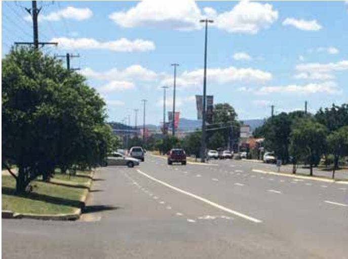
▲ THE ROAD IS A DIVIDED CARRIAGEWAY WITH A TURFED/TREED MEDIAN AND BIKE LANES ON EITHER SIDE
