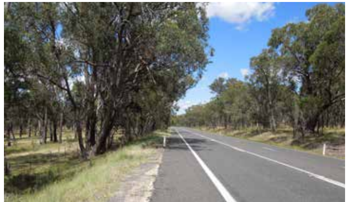
▲ TYPICAL OPEN WOODLANDS ADJACENT TO THE NEW ENGLAND HIGHWAY AROUND URALLA.
