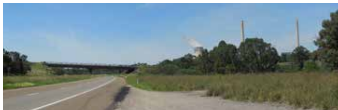
▲ BAYSWATER POWER STATION VISIBLE FROM THE HIGHWAY.
