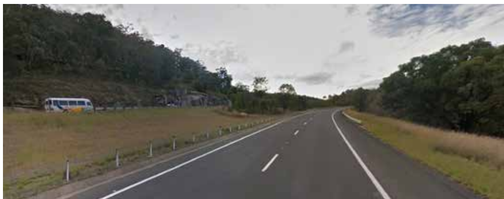
> INDEPENDENTLY GRADED CARRIAGEWAY NORTH OF MURRURUNDI INTEGRATES THE HIGHWAY INTO THE SURROUNDING LANDFORM (IMAGE CREDIT: GOOGLE)
