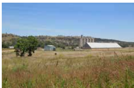
▲ GRAIN LOADING FACILITY NORTH OF MURRURUNDI
