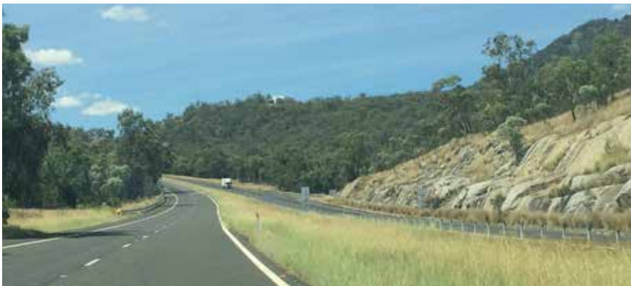
◀ MEDIAN AT MOONBI PROVIDES AN ENHANCED VISUAL OUTCOME AND BREAKS DOWN THE SCALE OF THE HIGHWAY
