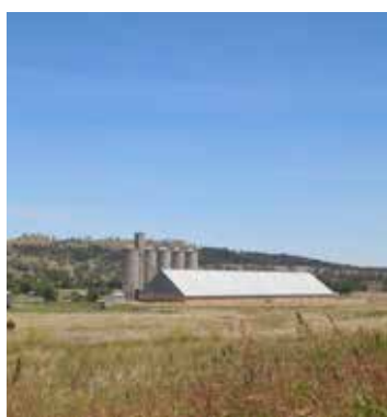
▲ GRAIN LOADING FACILITY NORTH OF MURRURUNDI
