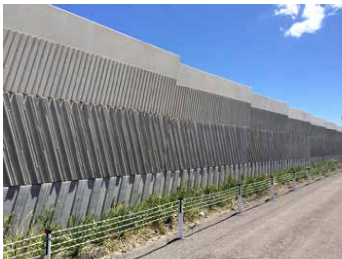
▲ HUNTER EXPRESSWAY NOISE WALL PATTERNING REFERENCES THE ADJACENT VINEYARD CONTEXT
