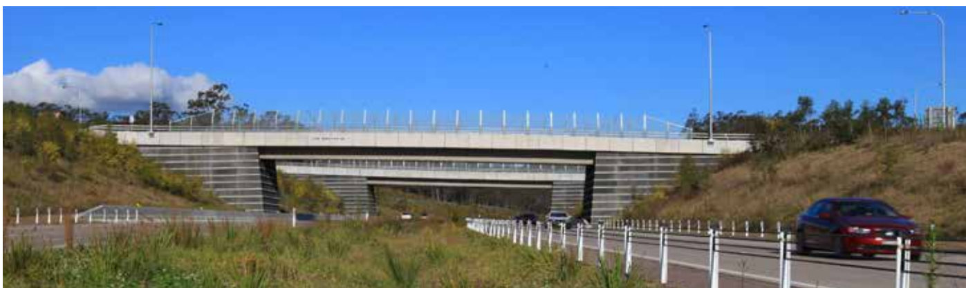
▲ WALLED ABUTMENTS ON THE HUNTER EXPRESSWAY
