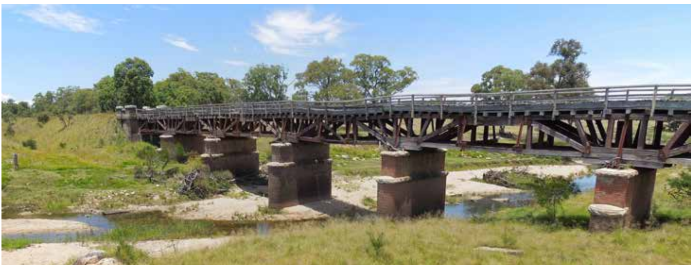
▲ HERITAGE RAIL BRIDGES VISIBLE FROM THE NEW ENGLAND HIGHWAY
