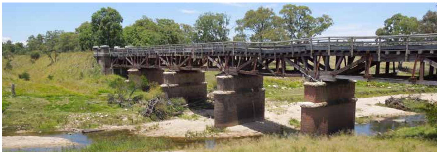
▲ TENTERFIELD CREEK RAIL BRIDGE
