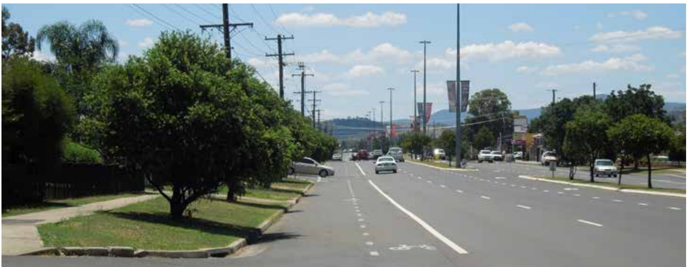
▲ TAMWORTH TOWN CENTRE - THE HIGHWAY INCLUDES A PLANTED MEDIAN AND VERGES, PARKING LANE AND CYCLE PATHS
