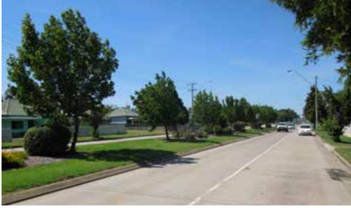
▲ PLANTED MEDIAN IN CORRIDOR THROUGH GLEN INNES.
