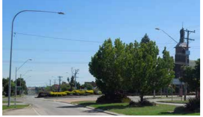
▲ PLANTED ROUNDABOUT AT INTERSECTION OF NEW ENGLAND HIGHWAY AND GWYDIR HIGHWAY.
