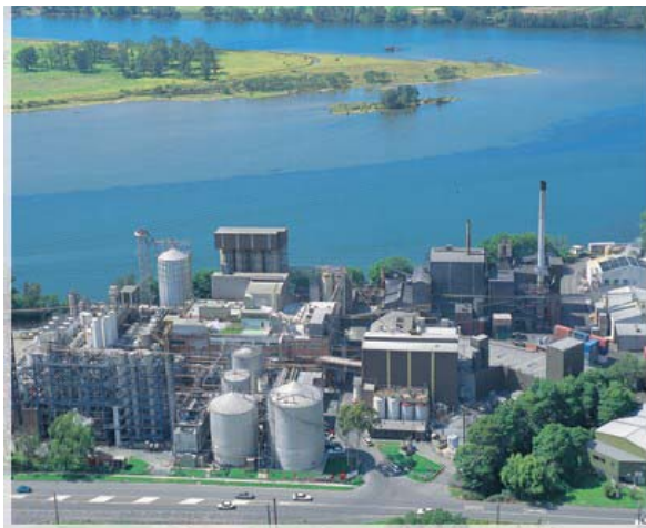
Figure 70 – Manildra's Bomaderry production facility
