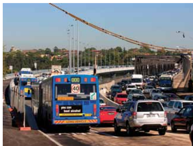
The completed $175 million Inner West Busway, January 2011.
