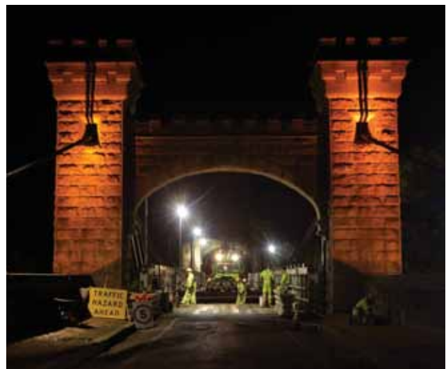
Maintenance work on Hampden Bridge, Kangaroo Valley, June 2011.
