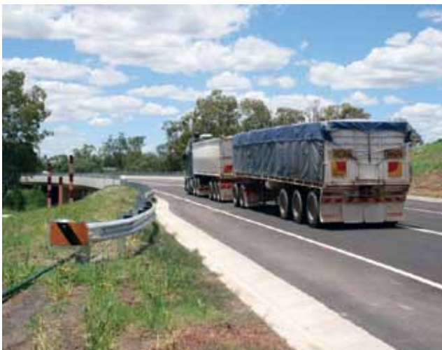
The completed Mehi River Bridge on the Moree Bypass, December 2010.
