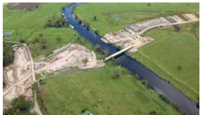
Aerial view of the temporary Myall River Bridge and new bridge works, Bulahdelah Bypass, January 2011.
