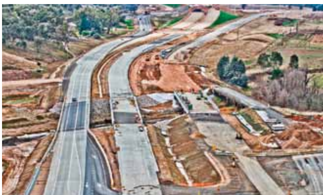
Aerial view of the Tarcutta Bypass, June 2011.
