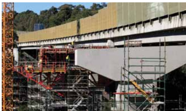
Terry's Creek upgrade, part of the M2 widening project, in construction, June 2011.
