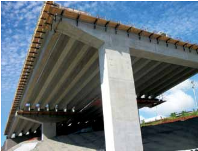
First span of super-T girders erected for the southern valley viaduct, Banora Point, May 2011.
