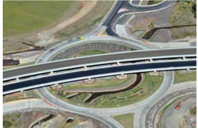
Teven interchange on the Ballina Bypass, May 2011.
