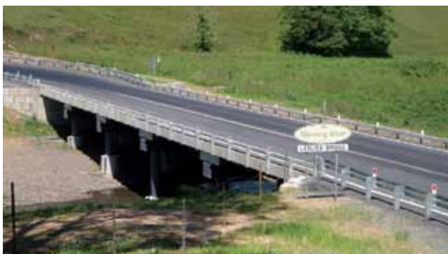
New Leslie Bridge, Manning River, completed under the Timber Bridge Partnership, December 2010.
