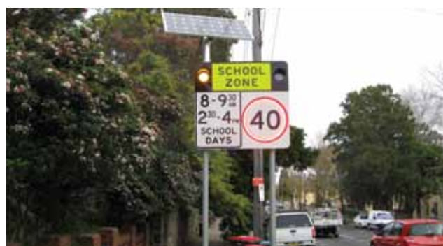
School zone flashing lights on Carrington Road at Waverley Catholic College, upgraded June 2011.
