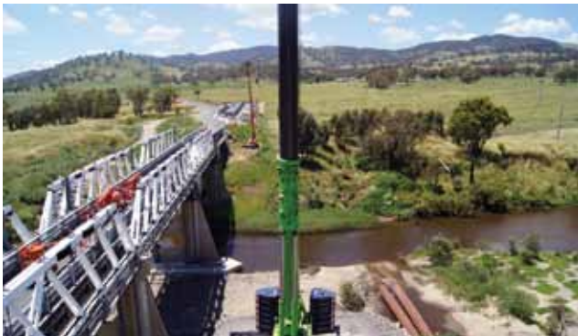
Restoration of the heritage-listed Tharwa Bridge, November 2010.
