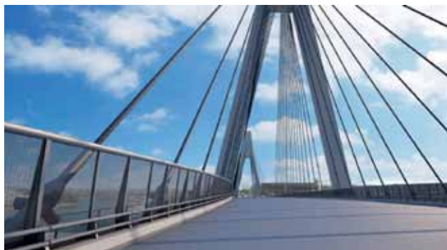
Urban design in the development phase: photomontage illustrating the visual impact of the proposed fence types on Anzac Bridge.
