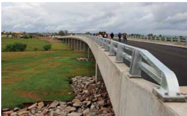
The completed Third Crossing of the Hunter River at Maitland, including the Harry Boyle Bridge, December 2010.
