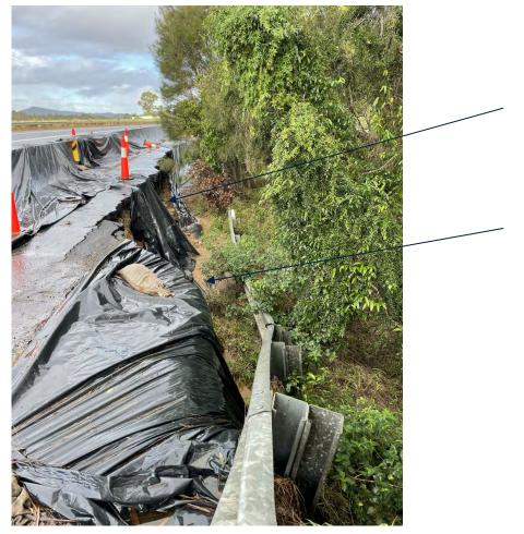
Recent slumping of headscarp pavement and fill materials. Regression back beneath pavement.
