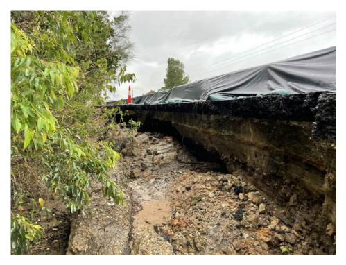
Photograph 3: 11 March 2021 - Headscarp exposing pavement layers and undercutting.
