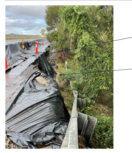
Slumping of headscarp pavement and fill materials. Regression back beneath pavement.
