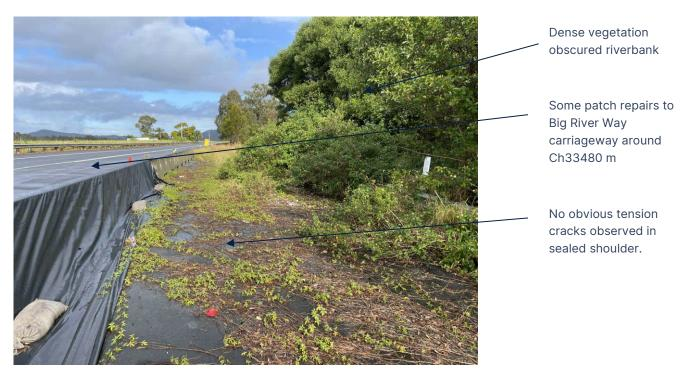
Photograph 4: 29 June 2021 - Ch33490 m - view south; wide sealed shoulder at southern end of slip.
