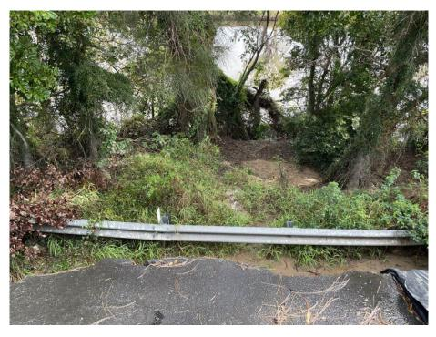
Photograph 8: 29 June 2021 - ~Ch33515 - view of slumped road embankment and riverbank below headscarp.
