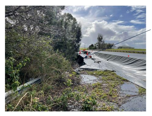
Slip headscarp with some slumping observed regressing back beneath pavement
