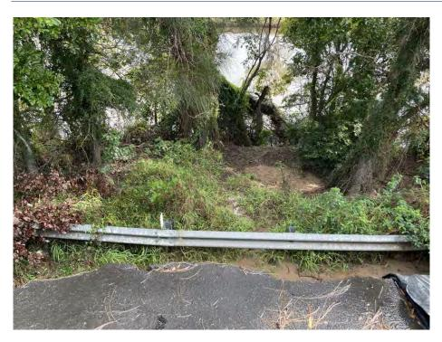
Photograph 4: ~Ch33515 - view of slumped road embankment and riverbank below headscarp.
