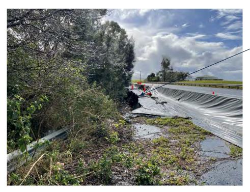
Landslip headscarp with some slumping observed regressing back beneath pavement
