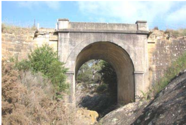
Black Bobs Creek Bridge, old Hume Highway alignment. Unreinforced concrete arch
