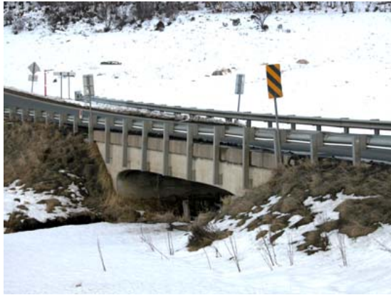
Diggers Creek (RTA Bridge No 6201) Simple curved soffit
