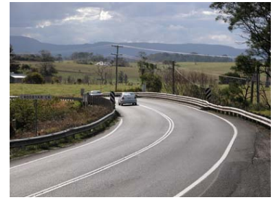
Croobyar Creek Bridge (RTA Bridge No 730) Retrofitted Thierail guardrailing
