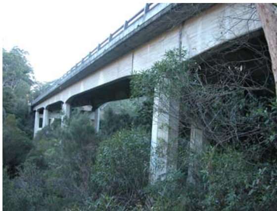
Woronora River (RTA Bridge No 152)
