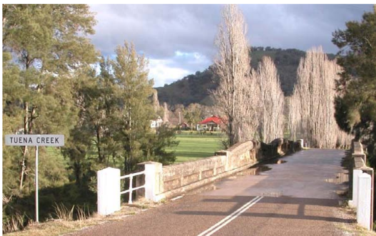
Tuena River (RTA Bridge No 6401)
