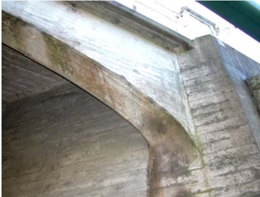
Middle Creek No 1 (RTA Bridge No 146) Complex shapes using timber formwork
