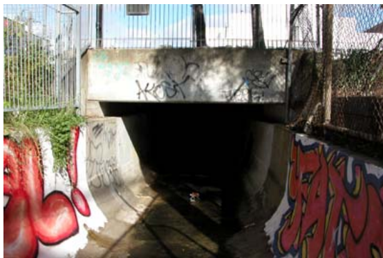
Entrance to culvert under Parramatta Road Burwood
