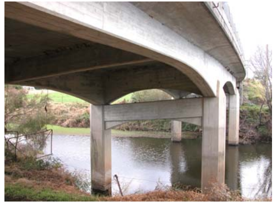
Croobyar Creek (RTA Bridge No 730) Complex curvature
