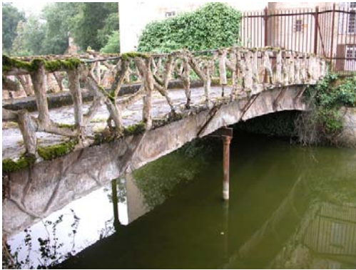
Bridge at Chateau de Chazelet, France (photos Sid French)
