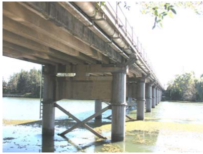
Hawkesbury River (RTA Bridge No 415) Cast iron caissons
