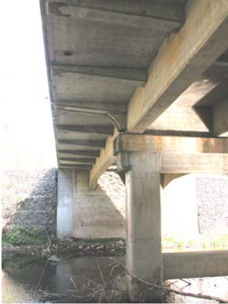
Broughton Creek Bridge (RTA Bridge No 704) Widened two span bridge composite with abutment
