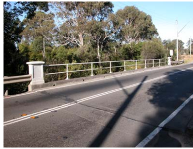
Harris Creek Bridge (RTA Bridge No 500) Pipe railings with concrete endposts
