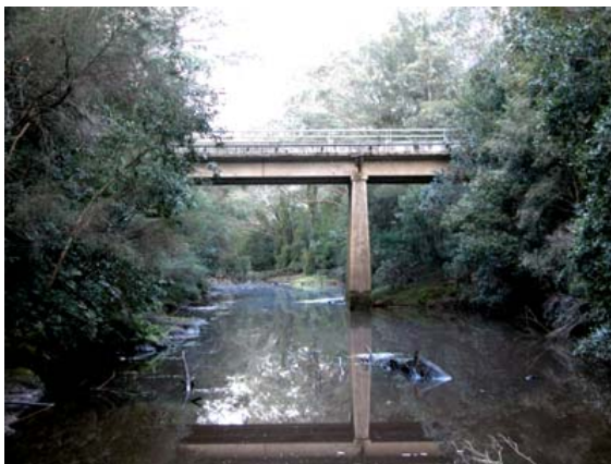
Wandandian Creek (RTA Bridge No 723) This sturdy high level structure was erected in 1929 replacing a set of three low level timber bridges vulnerable to flood. As well as motor traffic, the bridge was used by bullock teams dragging logs to the Wandandian Sawmill
