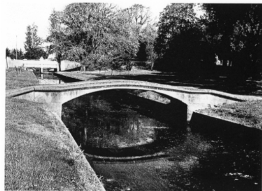
Otepunī Gardens footbridge c1899 (source Bridging the Gap by G Thornton)
