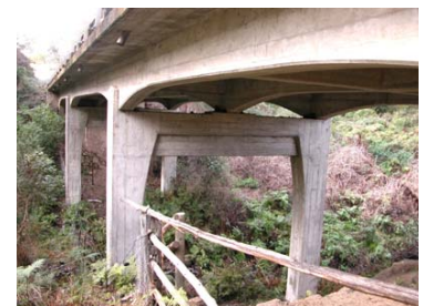
Couria Creek Bridge (RTA Bridge No 5978) Individualised pier framing
