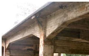
Wonboyn River Bridge (RTA Bridge No 6012) Bold straight and curved lines
