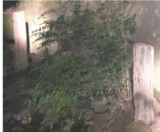
Middle Creek No 1 Remnant timber piles used for formwork support
