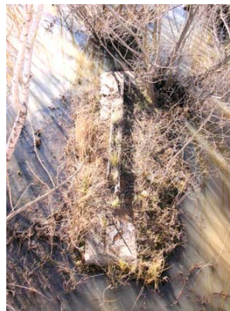
Concrete pier footing with base timber
