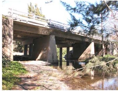
Yellow Rock Bridge (RTA Bridge No 790) Mass concrete wall piers
