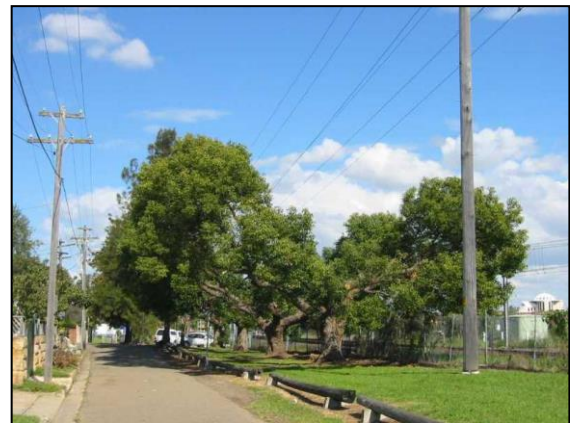
Figure 17. This tree at Belmore is continually pruned to achieve suitable clearance from the electrical feeder. This unsustainable and expensive situation could be solved by replacing the large trees with suitable vegetation in consultation with Local Council.
