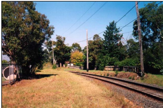
Figure 24. This stable Corridor on the Carlingford line is maintained by slashing. Any weed control should be undertaken using minimal impact techniques so as not to disturb the stable grass sward
