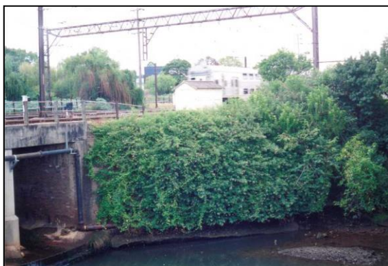
Figure 3. Weed infested rail corridors such as this one at Clyde, are difficult and expensive to maintain
