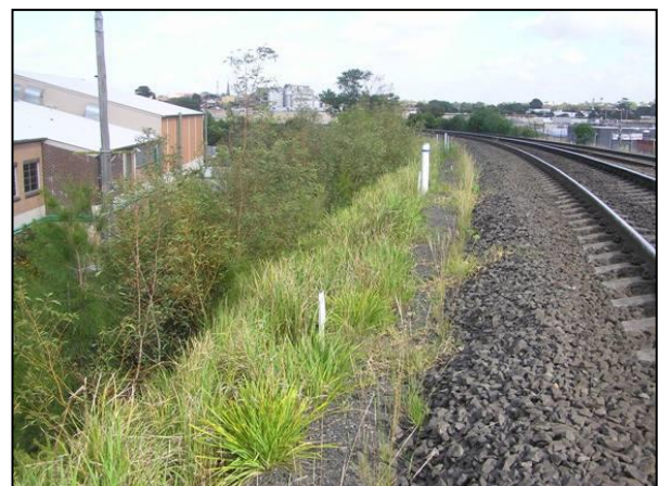
Figure 14. A previously weed infested embankment at Sydenham that has been revegetated with local indigenous plants, creating a low maintenance and aesthetically pleasing corridor.
