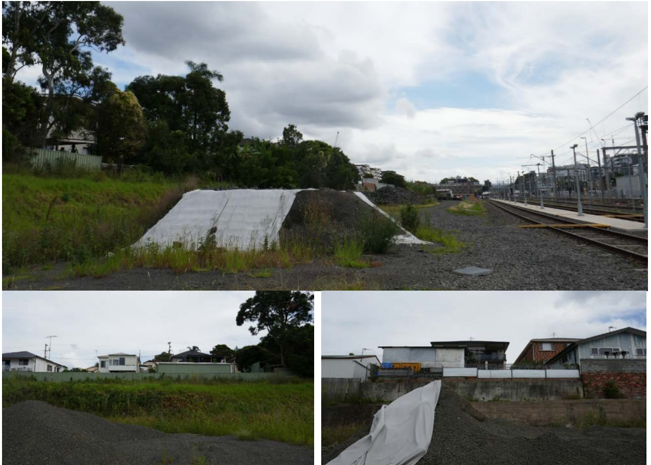
Figure 6-10: Boundary between Wollongong Stabling Yard and the rear of dwellings on Gladstone Avenue
