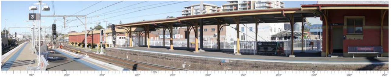
Figure 3-4: Wollongong Station – Existing view
