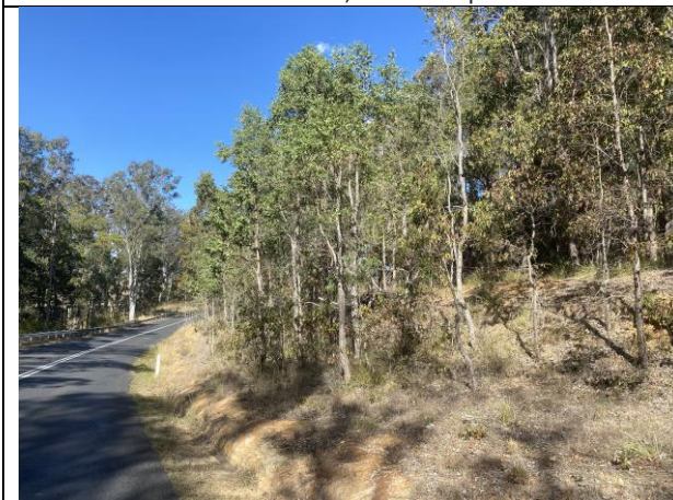
Plate 11: Regrowth Swamp Box and Broad-leaved Apple west of culvert in Plate 10 (ch. 49800); all trees within ~7m of the road (~ ch. 49820 -) 49850) to be removed.
