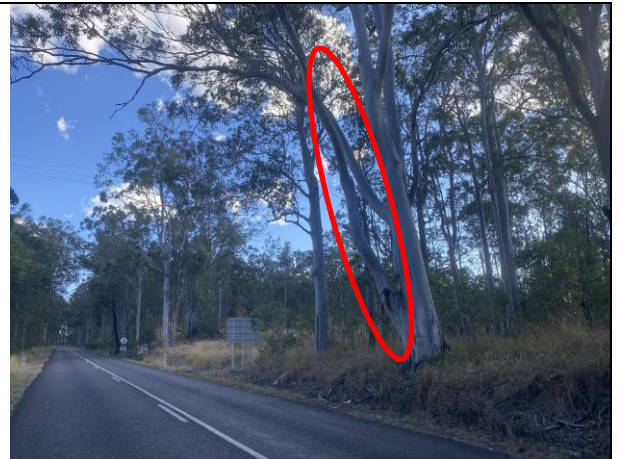
Plate 8: Mature Forest Red Gum west of Captains Creek – pruning of leaning limb (circled) required; tree retained.
