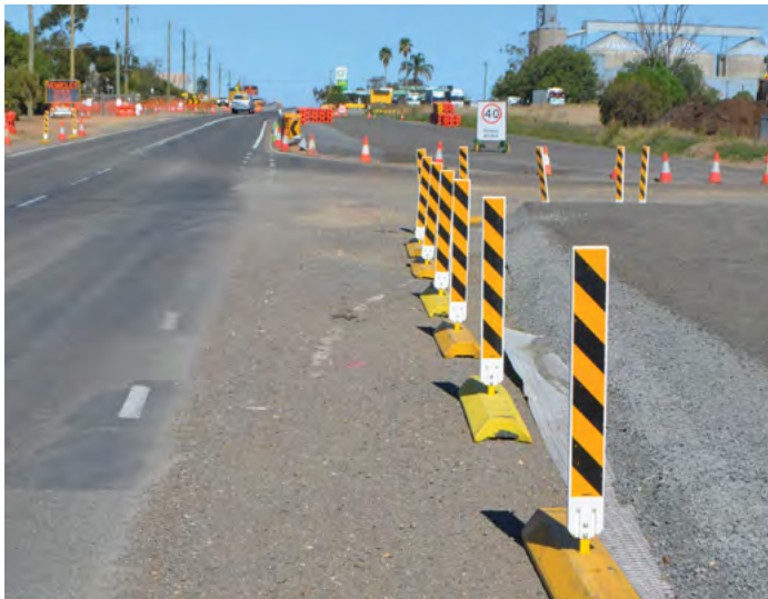
Pictured: Millie Road intersection upgrade in progress
