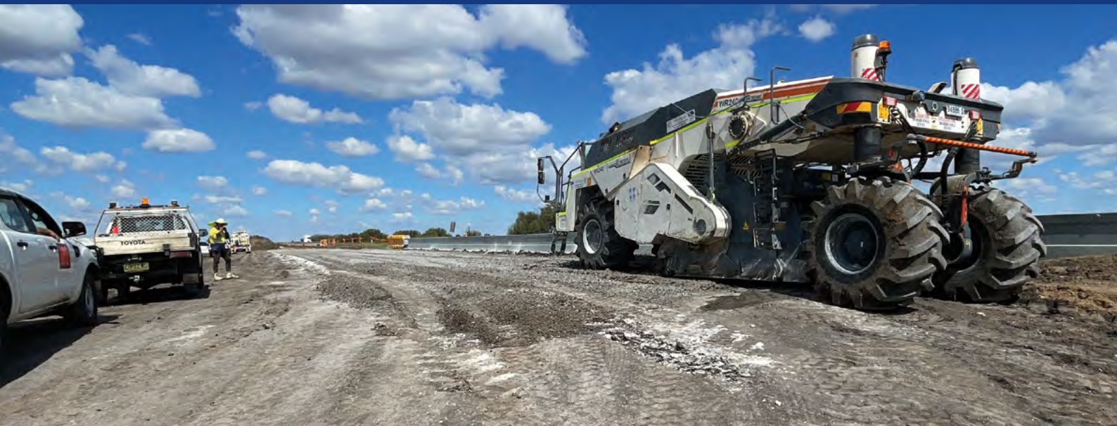
Pictured: Stabilisation works in progress in Section 5 near Moree
