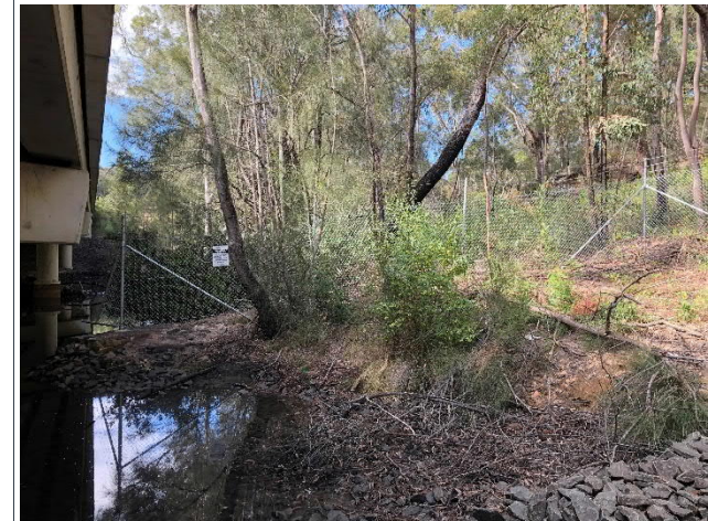
Photo 4.2 Newly installed Defence fence at Deadmans Creek. This may require modification or replacement for Option 2 to be effective. Image courtesy of TfNSW
