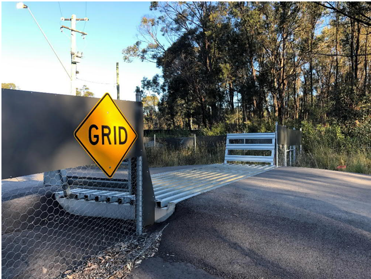
Photo 4.6 Example of a koala grid along Picton Road, where there is a break in continuous fencing for residential access
