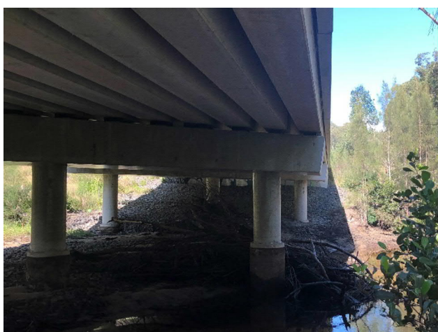
Photo 3.1 The multi-span concrete bridge that crosses Deadmans Creek (L) and the rip-rap scour protection that surrounds the bridge abutments and creek banks (R)
