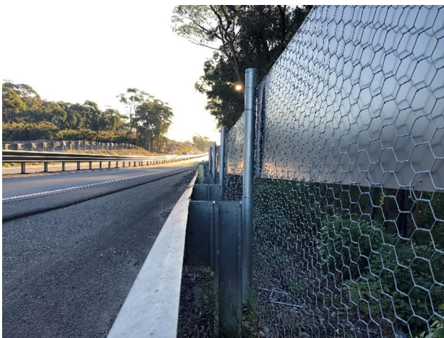
Photo 4.5 Example of koala fencing along Picton Road in Sydney's south-west. The photo on the right shows a break in koala fence to provide vehicle access. The gap underneath the gate is ~500 mm, which fauna can easily navigate their way under. Gaps underneath gates need to be minimised as much as possible
