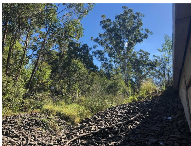
Photo 3.1 The multi-span concrete bridge that crosses Deadmans Creek (L) and the rip-rap scour protection that surrounds the bridge abutments and creek banks (R)
