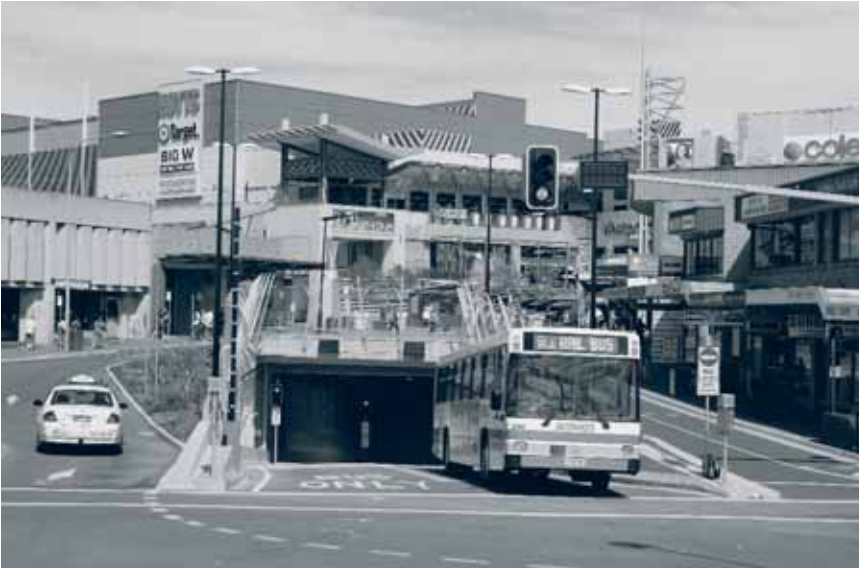
The Patrick Street bus tunnel in Blacktown, commissioned in April 2006, improves access for shoppers and bus travellers around a busy shopping complex.
