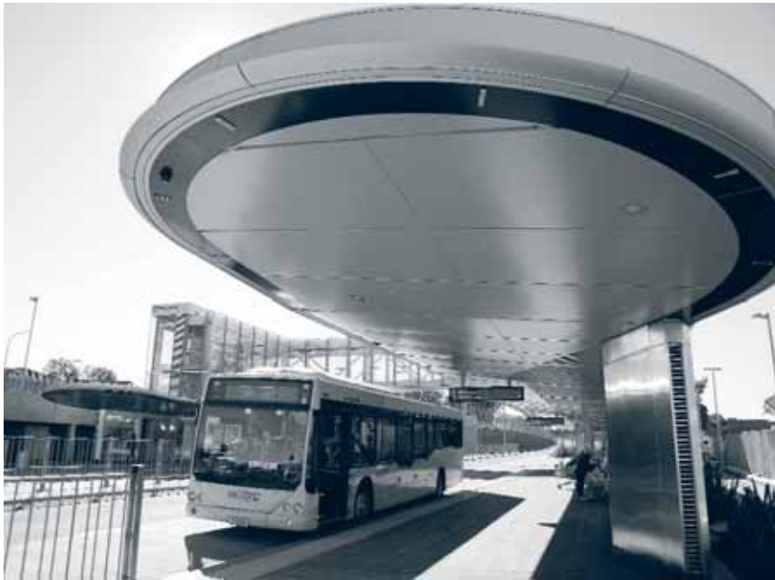
The Prairiewood Station on the Liverpool Parramatta T-way is part of a new public transport system for western Sydney.
