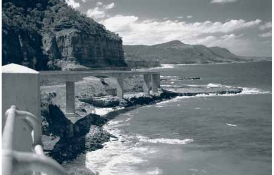
Sea Cliff Bridge on Lawrence Hargrave Drive, completed in December 2005, has received several awards for construction excellence.
