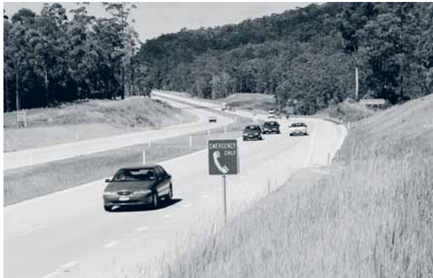
Dual carriageways on the Pacific Highway at Bulahdelah provide a new highway alignment that improves safety.
