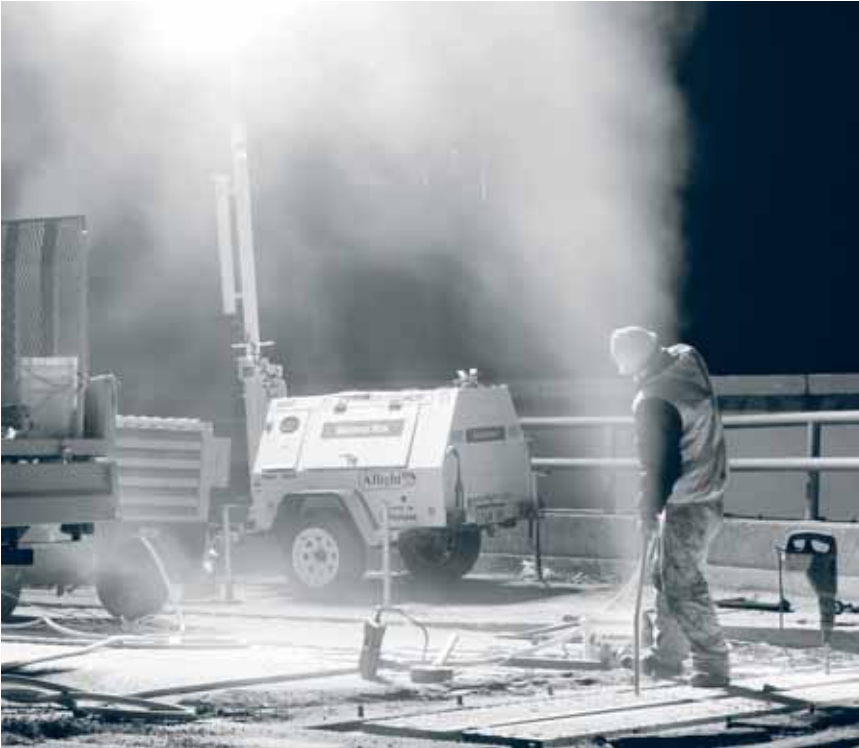
RTA Bridge Services – civil crew undertaking night works on the Cahill Expressway to replace expansion joints.
