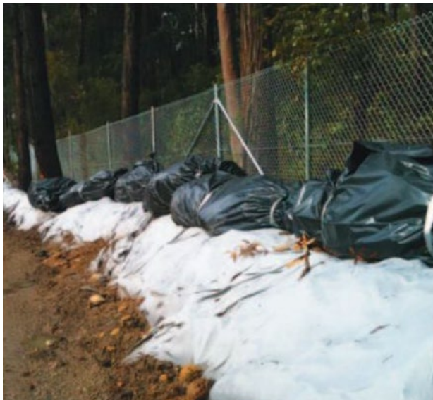
Figure 7.11: Removed vegetation was securely wrapped in black plastic bags before disposal to prevent the spread of the pathogen Myrtle rust on the M2 Upgrade, Sydney Region (Photo: Nicholas Francesconi, TfNSW).
