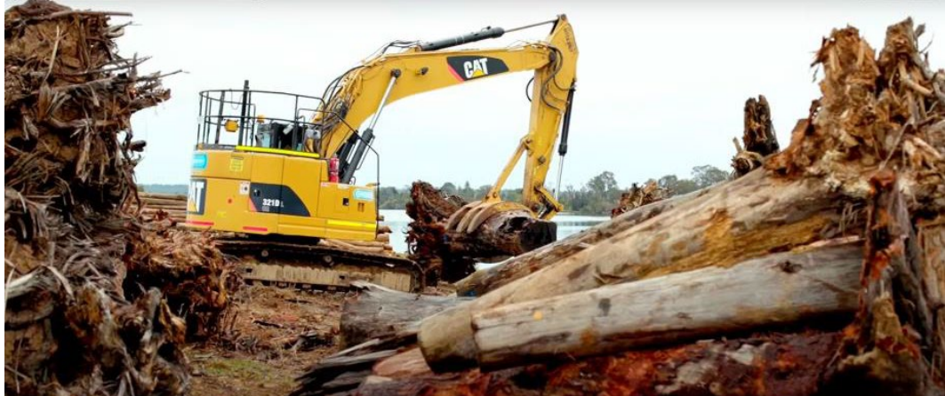
Figure 5.4: TfNSW provided 400 rootballs and logs felled for the Pacific Highway Upgrade for the Clarence River riparian rehabilitation project to stabilise the river banks and improve fish habitat (Photo: Soil Conservation Service).
