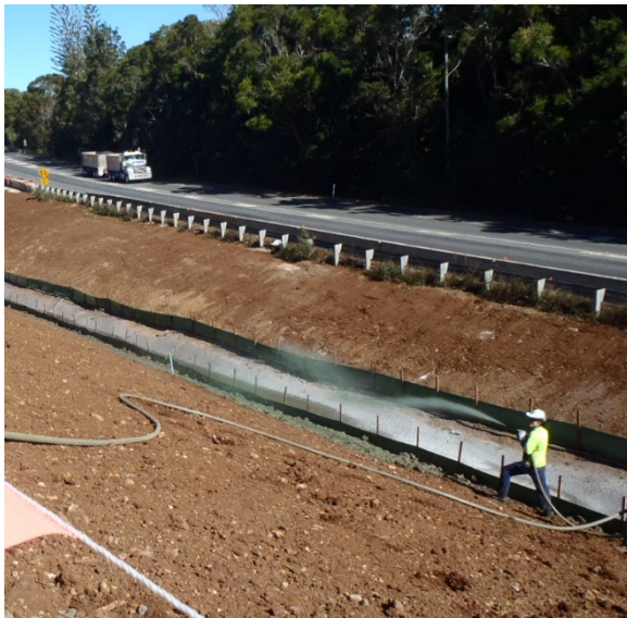
Figure 3.4: Hydroseed application on a prepared batter (Photo: TfNSW).
