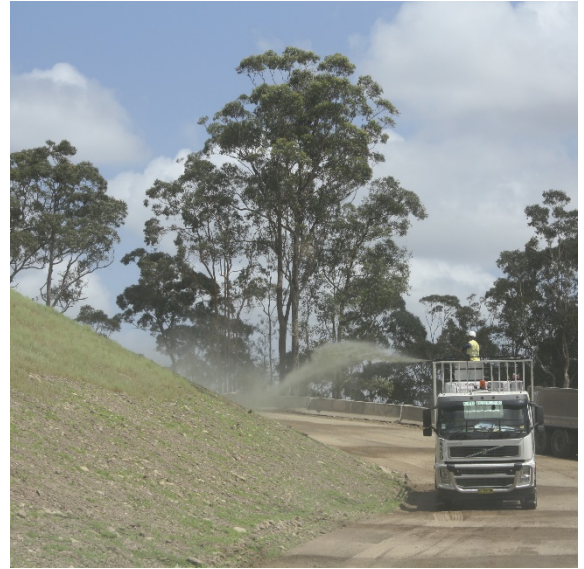
Figure 3.8: Hydromulch being sprayed on a batter on the Hunter Expressway (Photo: TfNSW).
