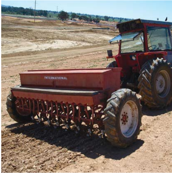
Figure 3.7: Direct seeding a batter (Photo: Martin Sullivan, TfNSW).
