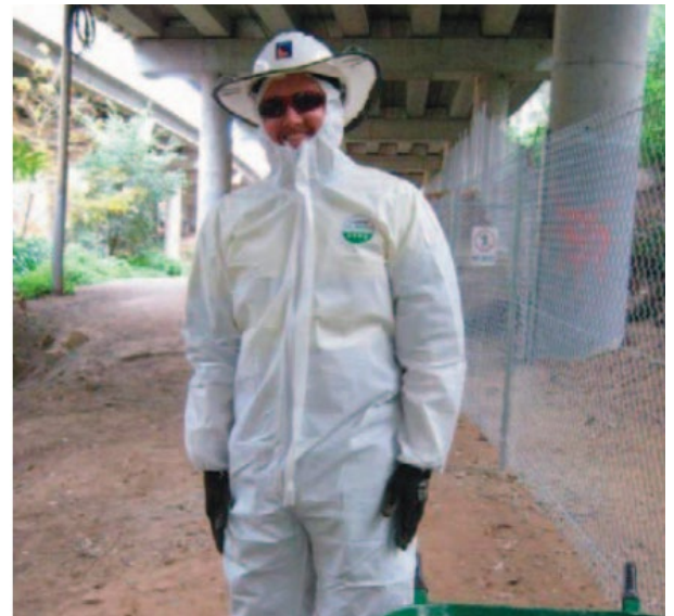
Figure 7.12: Disposable suits worn on the M2 Upgrade (Sydney Region) following Myrtle rust identification adjacent to Blue Gum High Forest critically endangered ecological community (CEEC). This level of hygiene is recommended when working in Myrtle rust sites that are adjacent to highly sensitive ecological areas (Photo: Donald Cheong, TfNSW).
