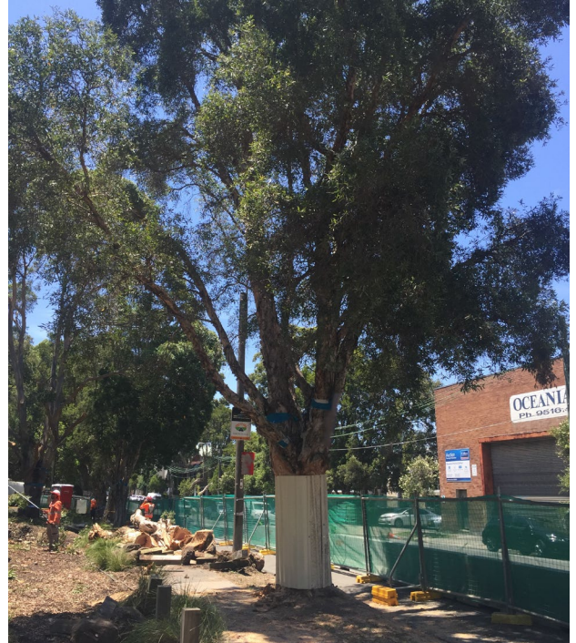
Figure 1.6: Tree-guards can be installed on trees during the pre-clearing process to prevent climbing animals being present during clearing (Photo: Brenton Hays, TfNSW)
