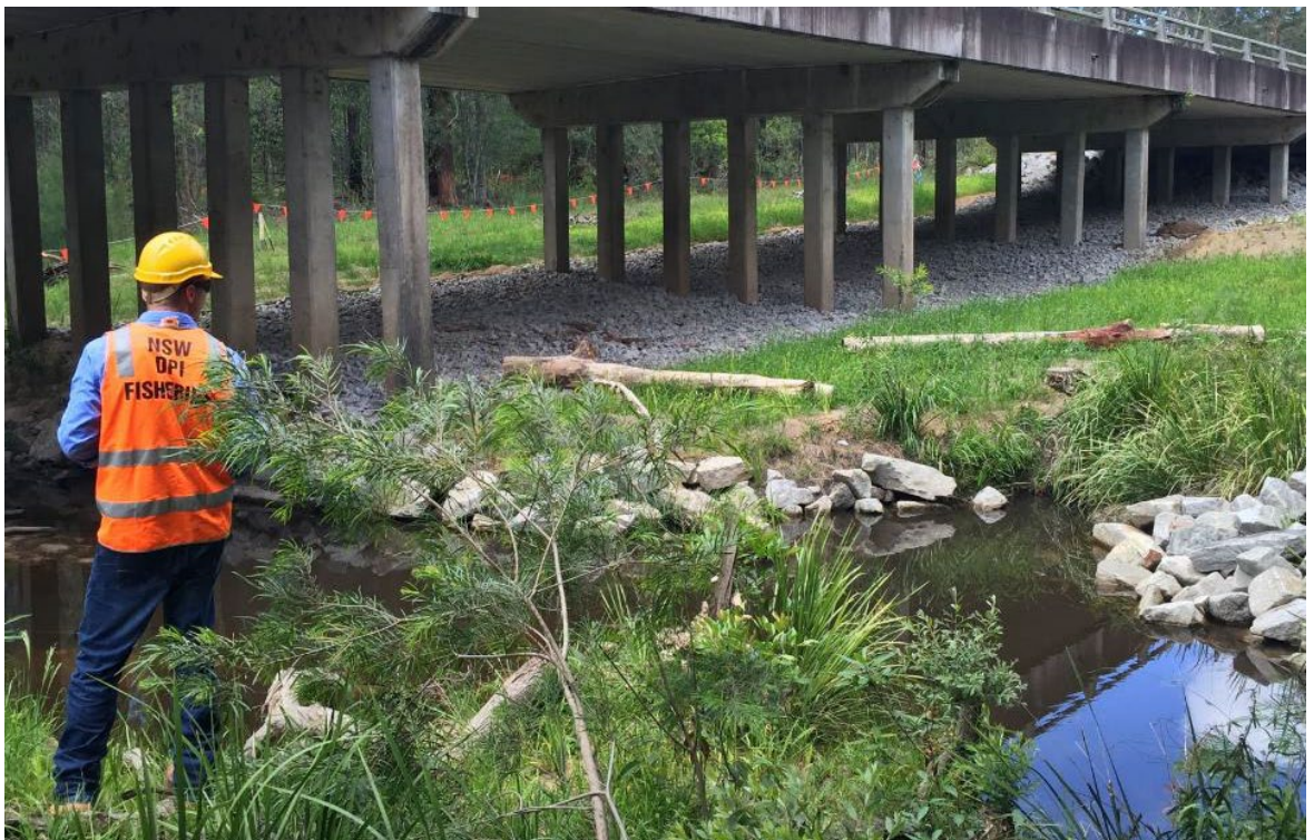
Figure 10.1: Even disturbed aquatic habitat and riparian zones can provide important resources for flora and fauna. This waterway on the Woolgoolga to Ballina Pacific Highway Upgrade Project is being inspected by a DPI Fisheries officer (Photo: Anthony Arena, TfNSW).
