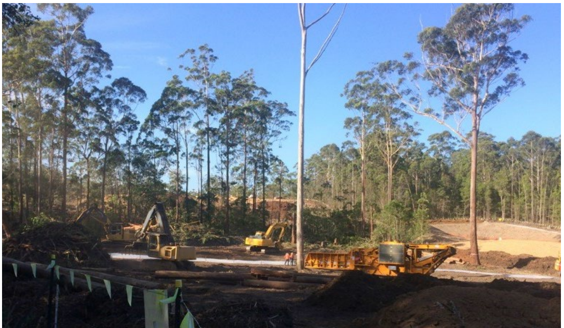
Figure 4.2: Staged habitat removal taking place for Nambucca Heads to Urunga Pacific Highway Upgrade to minimise impacts on biodiversity (Photo: Sandpiper Ecological Surveys).
