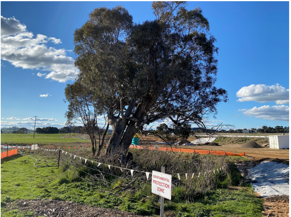
Figure 2.9: An example of tree protection using flagging on Barton Highway project (Photo: Amy Evans, TfNSW).
