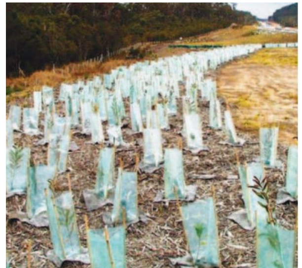
Figure 3.10: Planting with a diverse range of species that are representative of the nearby vegetation communities around the Pacific Highway at Karuah (Photo: Paul Murray, TfNSW).
