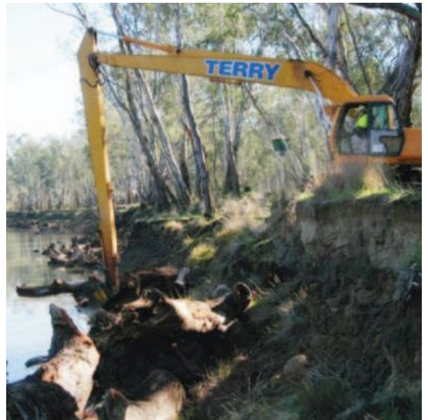
Figure 10.3: Snag timber from the Hume Highway Duplication project was placed in the Murray River and now provides habitat for threatened native fish species such as Murray Cod ( Maccullochella peelii peelii ) and Trout Cod ( Maccullochella macquariensis ) (Photo: J Fredrickson, DPI).
