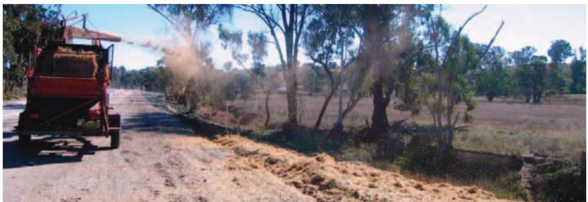
Figure 3.6: Straw mulching over a hydroseeded embankment. A tackifier (adhesive) is sprayed over the straw to bind it in place. The materials used must be appropriate to the local context, and consider fire risk, high wind and erosion profiles (Photo: Leigh Trevitt, TfNSW).
