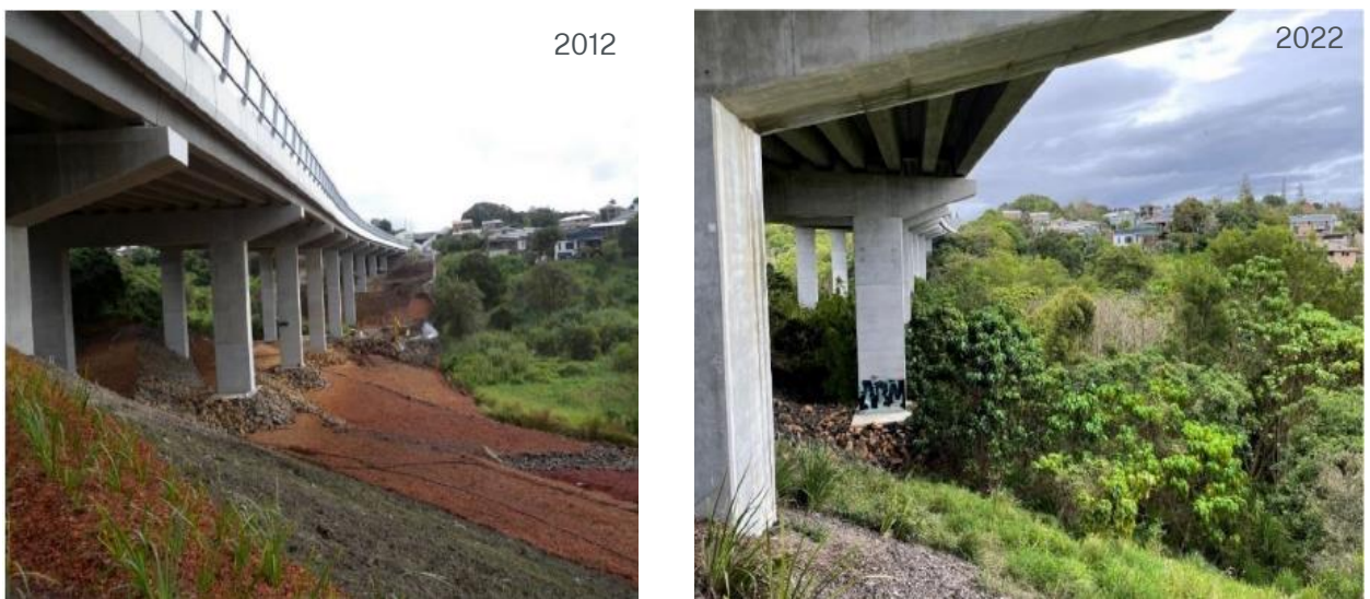
Figure 3.11: Ten years of rainforest revegetation, Banora Point Upgrade of the Pacific Highway. Photo on left taken post construction in 2012. Photo on right taken in 2022 showing progress over 10 year period (Photo: Alex Nicol, TfNSW).
