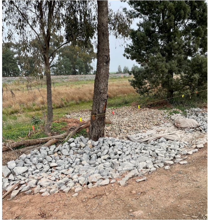
Figure 2.13: An example of poor practice. Construction materials should not be piled against trees and should be located outside the tree protection zone (Photo: Mel Cotterill, TfNSW).
